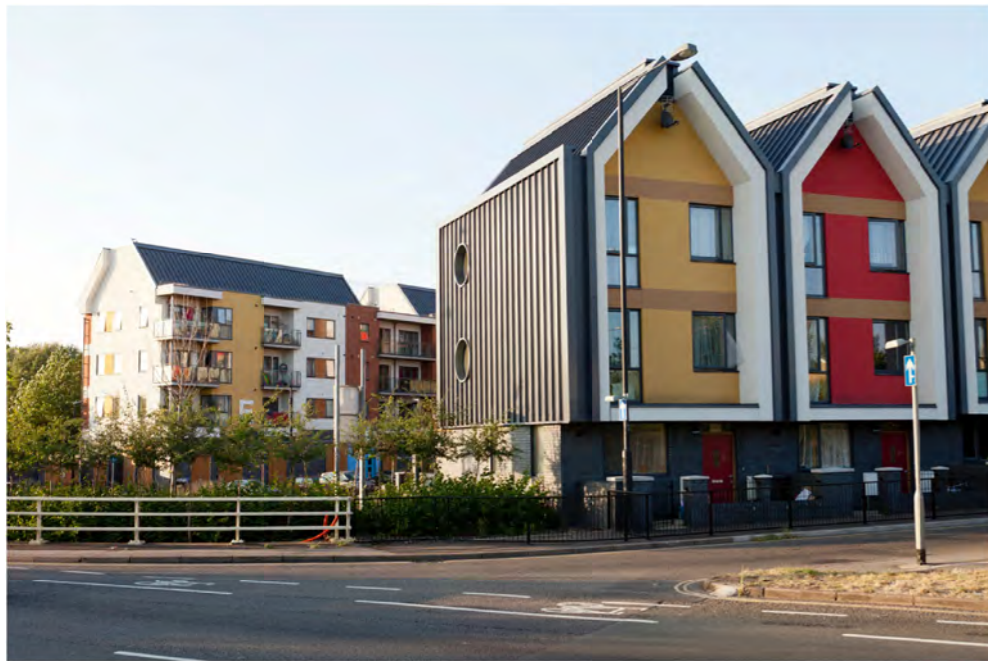
The recent J3 Development at junction 3 of the M32 provides an element of residential accommodation adjacent to the M32. This development features metal standing seam cladding on the roof and some of the external walls. The development also features bright colours which provide the scheme with vitality and make it easily recognisable.
