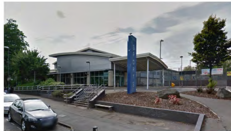
This sports centre is a dynamic building with an expressive roof, the building is largely clad with metal panels
