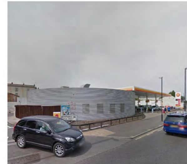
The shell garage features a distinctive curved metal wall
